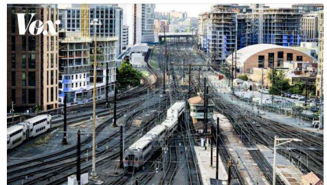
The Union Station train depot in Washington, DC. The US is the sixth-most expensive country in the world in which to build rapid-rail transit infrastructure. | Stefani Reynolds/Bloomberg via Getty Images
